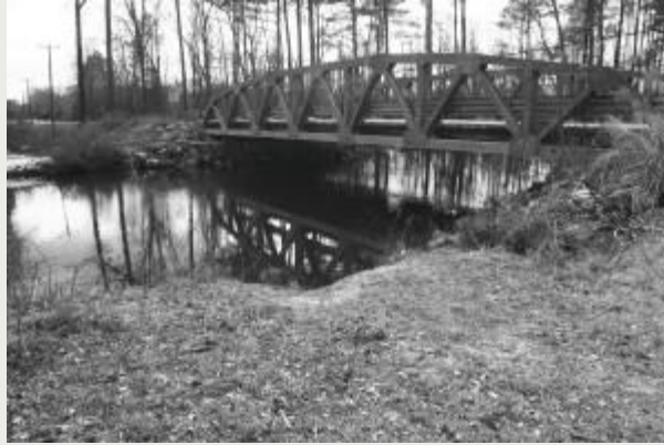
Site of Stuart's bridge rebuilding to cross Chickahominy River. photo by Randall flynn
